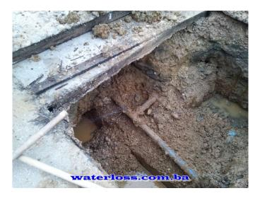
In the frame of Water loss reduction project in the five municipalities in Middle Bosnia from 12.11.2012. started sound leak dection action in DMA Mahala in Vitez municipality. At the beginning of this action 3 large underground leaks were detected, which the employees waterworks in Vitez repaired immediately.
